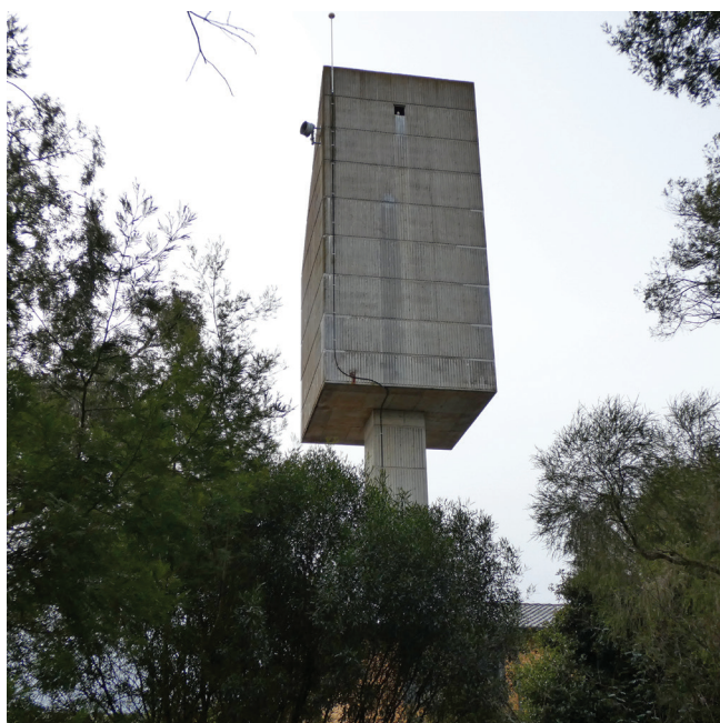
Figure 1. The water tower showing the entrance to the nest-box near the top and a male falcon on the ledge of the nest-box.
