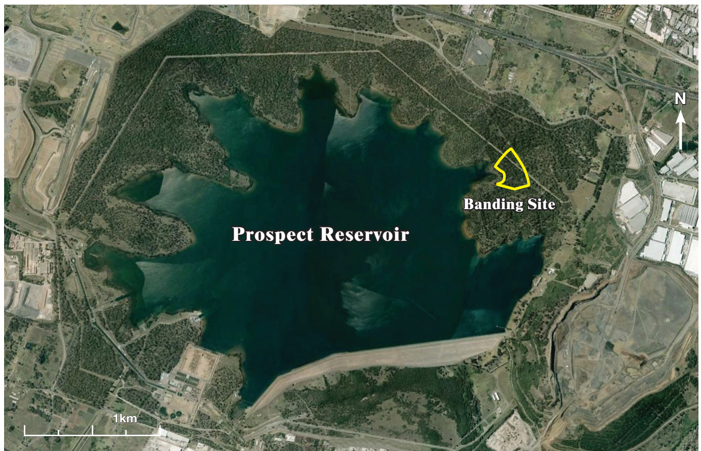
Figure 1. Banding Site Prospect Reservoir.
